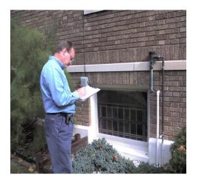
Inspector is recording an installed Pressure Vacuum Breaker. This device is testable and is typically installed on underground irrigations systems that are connected directly to the city water supply.
