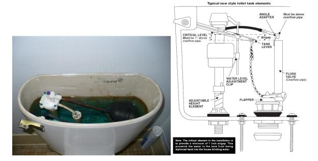
Older toilets are often equipped with fill valves that are submerged below the water level. Installing a new Anti-Siphon Ball Cock Assembly will fix the problem. These valves are inexpensive and are available at Home Depot, Lowes, or your local hardware store.
