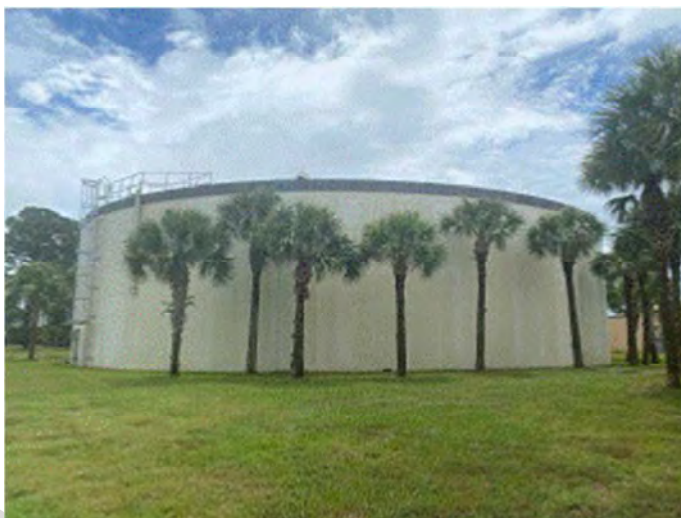
R Photo No. 10. Ground Storage Tank
