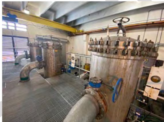
SLWSD ROWTP Micro Cartridge Filter
