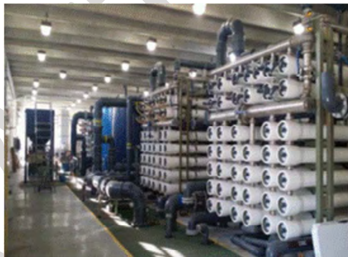
Reverse Osmosis Membrane Treatment Systems
