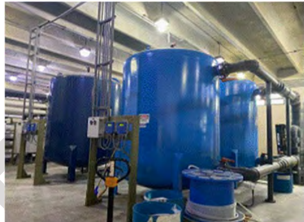
ROWTP Calcite Contactors
