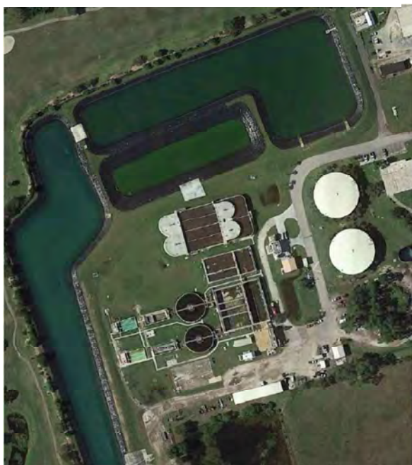
FIGURE 5. SLWSD WWTP (AERIAL VIEW)
