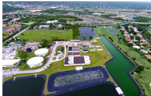
SLWSD WWTP (AERIAL VIEW)
